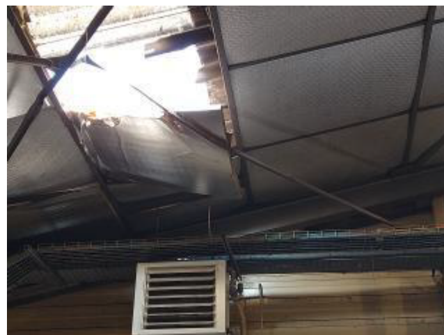
Figure 5 : Plafond perforé
